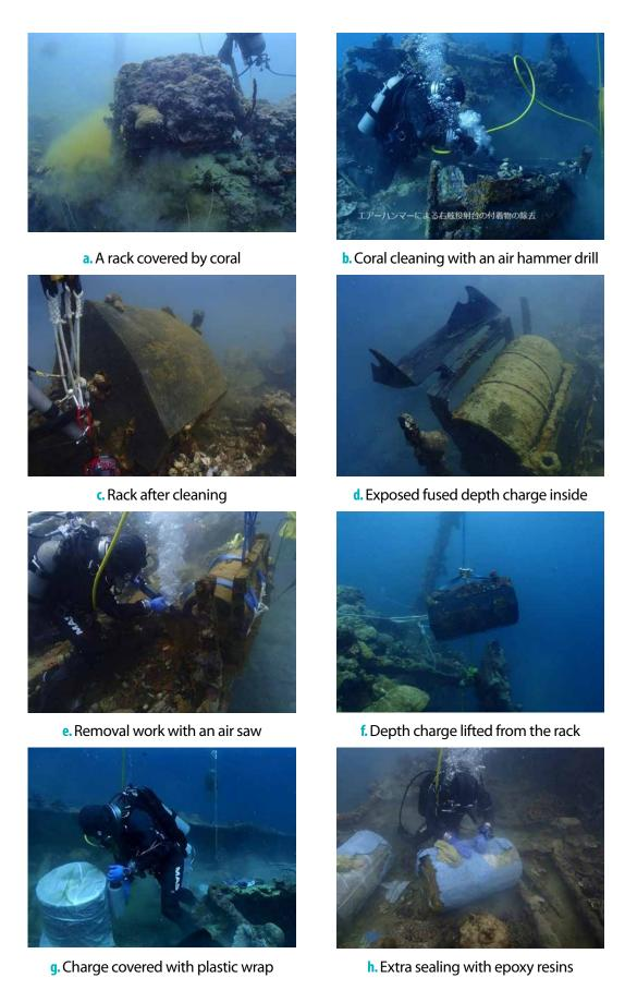
Figure 2-4. Removal process for fused depth charges ©JMAS/Palau HPO
