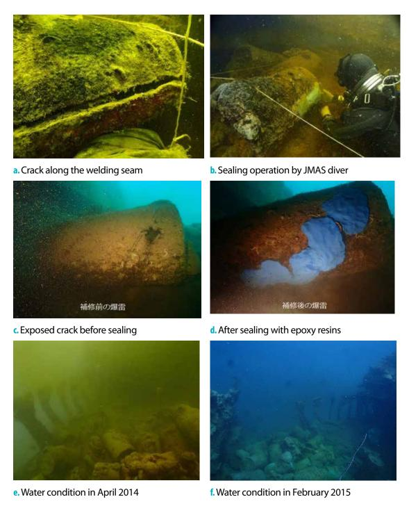
Figure 2-3. Sealing operations at the Helmet Wreck site. ©JMAS/ Palau HPO
